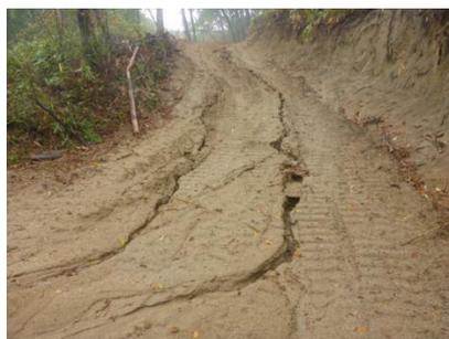
**Figure 1.** Operation road where the surface was eroded
