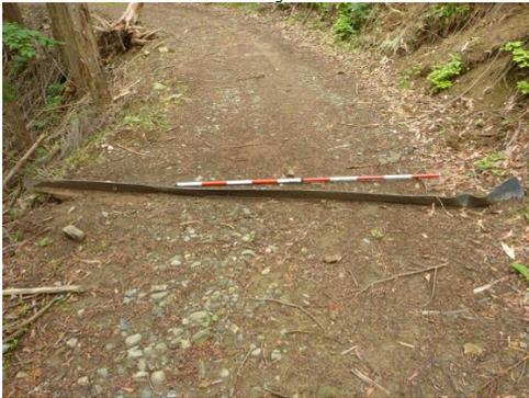
Figure 2 Rubber cross drain
