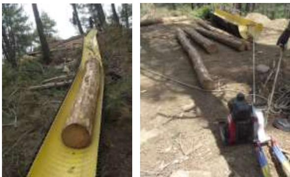
Figure 2. Pulling of the Wood-Based Products at Uphill Slope by Mobile Winch
