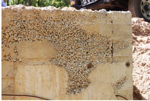
Figure 2. The used deficient materials
