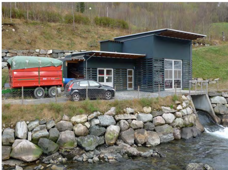
Vallestadfossen power station 1 MW
