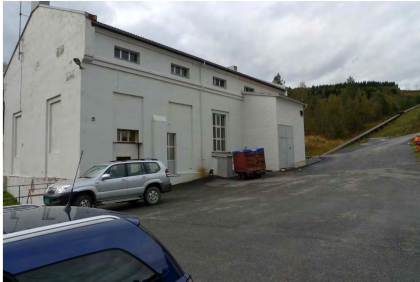
Istad power station 2.2 MW
