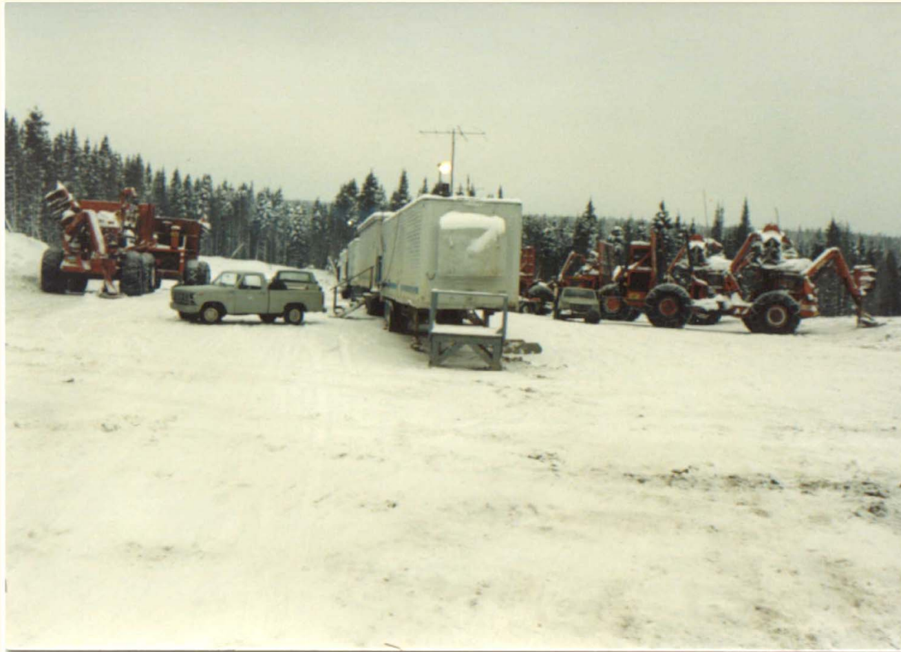
The support crew.
