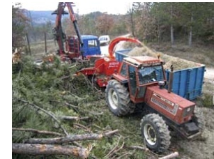
Chipping at the road side
