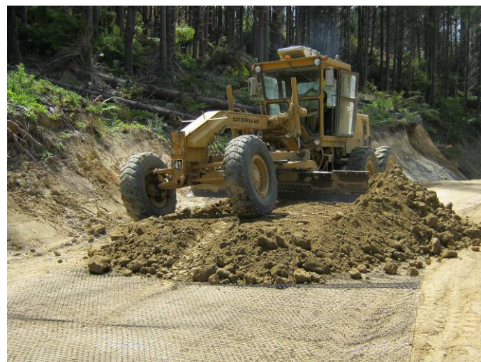
Figure 8: Spreading using a grader over geogrid.
