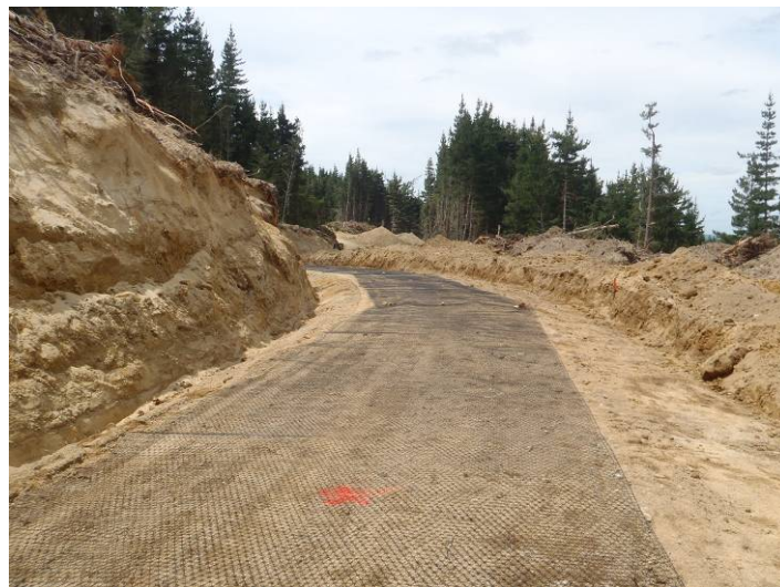
Figure 3: Geogrid is used in a curve on a forest road.
