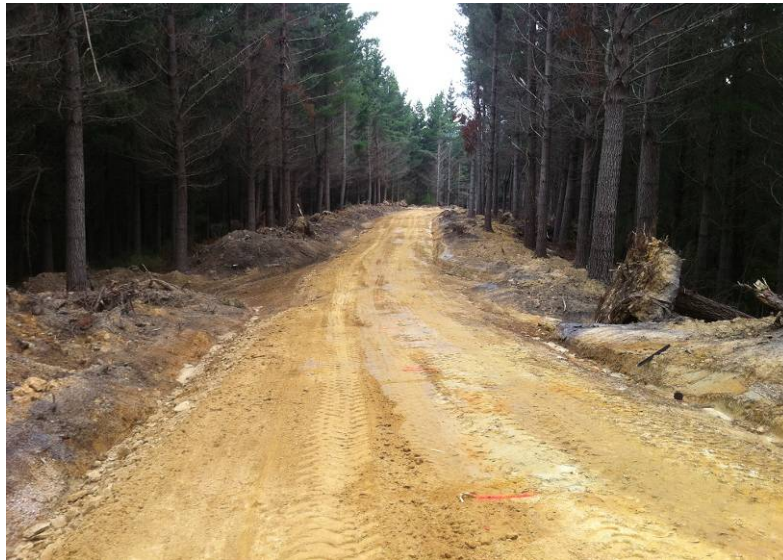
Figure 5: While the subgrade may look uniform, geotechnical testing, such as CBR measurements and or soil plasticity tests often indicate that forest road subgrades vary significantly over relatively short stretches, making exact design difficult.
