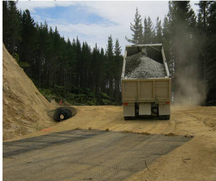
Figure 7: Covering Geogrid using a dump truck.
