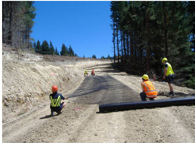
Figure 2: Placing a 25 meter section of geogrid into position
