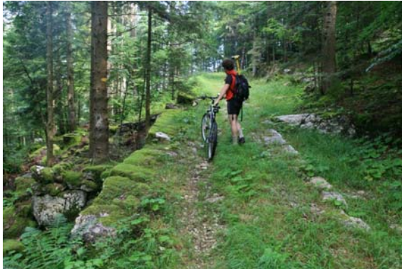
Figure 4: Evaluation on the deterioration of retaining walls
