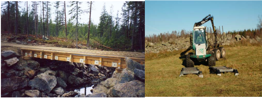
Figure 1. Bridges for crossings from left to right, semi fixed (Martinsons, http://www.martinsons.se ) and Hulttins temporary steel bridge ( http://www.hultdins.se/swe/index.htm ). Photo Martinsons (left) Eva Ring (right).
