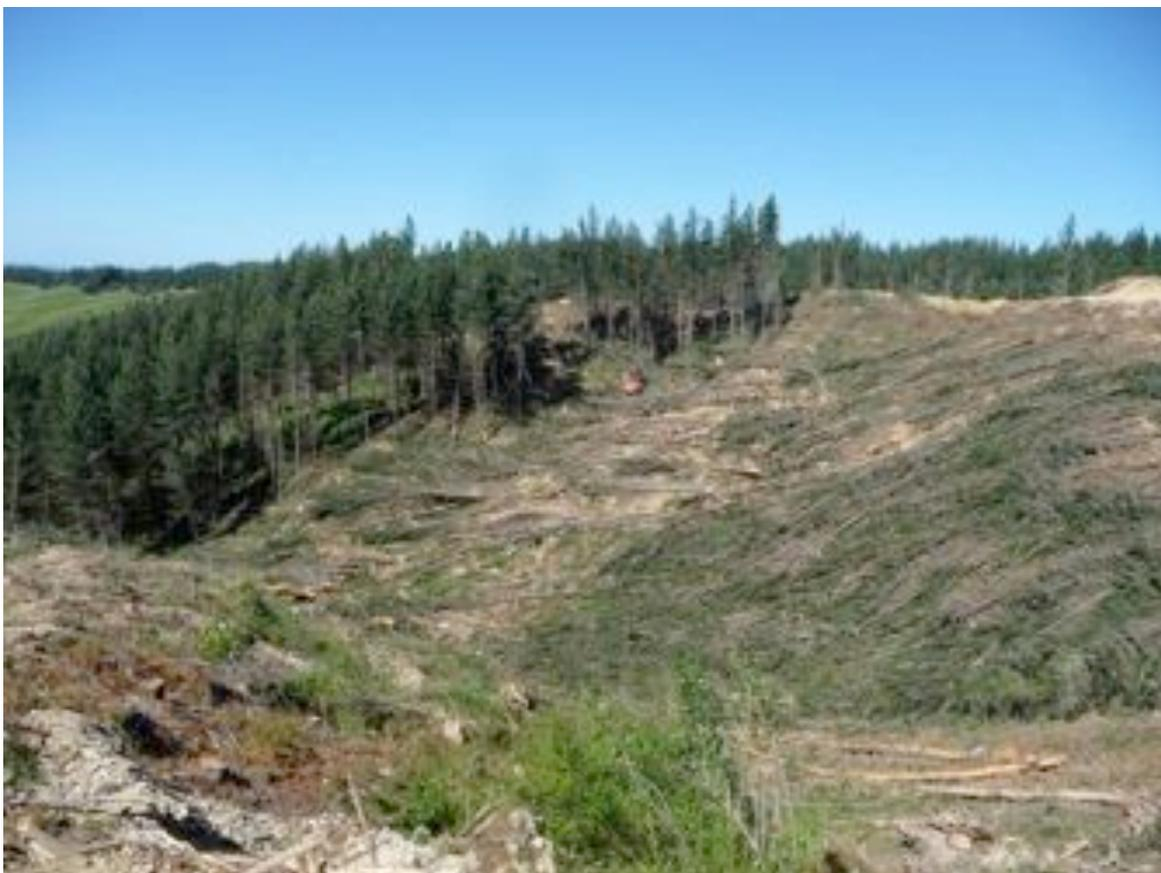
**Figure 4.** Feller-director felled and bunched trees laid on the slope on the left and handfelled trees can be seen on the right of the photograph, below the hauler pad (Kelly Logging Ltd).
