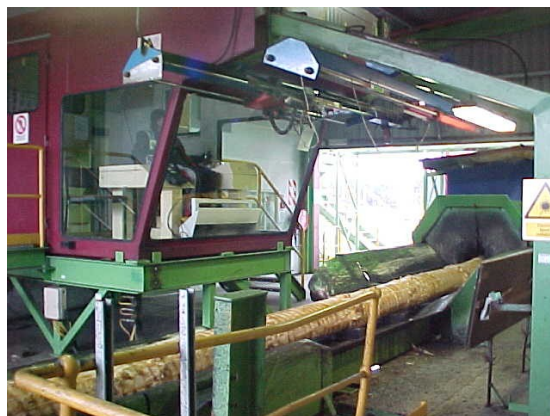
Figure 2: Grading operator booth at the KPP.
