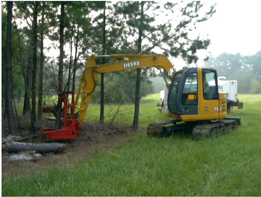
Figure 1: Small excavator with bunching shear head (John Deere 75C)
