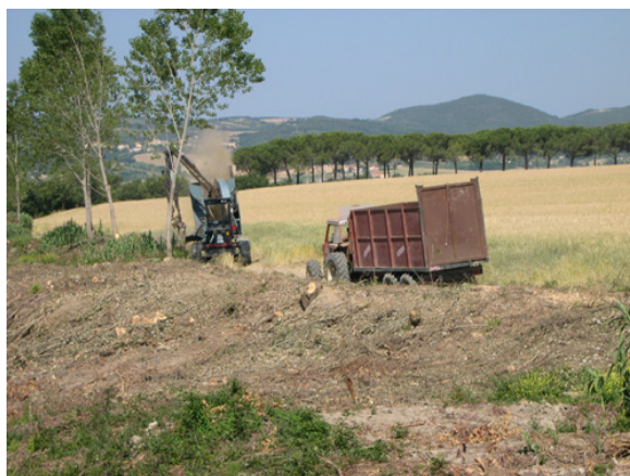
Figure 3: Santa Luce (PI) - vegetation clear-cut and chipping of the river’s “Fine” banks
